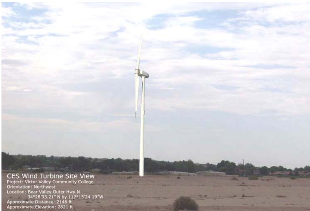
Figure 6. View of Proposed Wind Turbine from Bear Valley Road (looking northwest)
