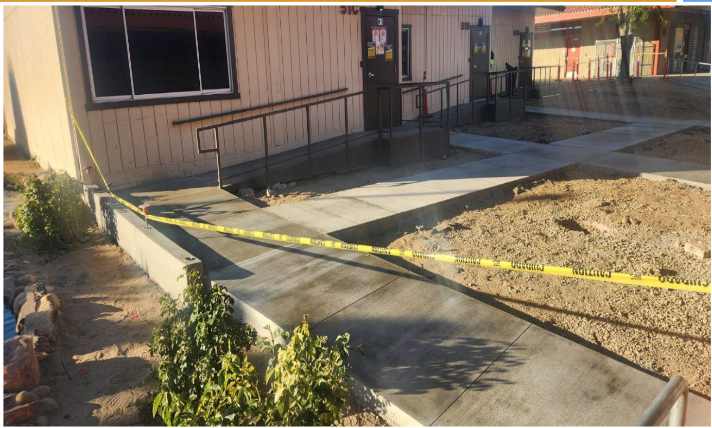
New concrete ramps for Bldg. 51
