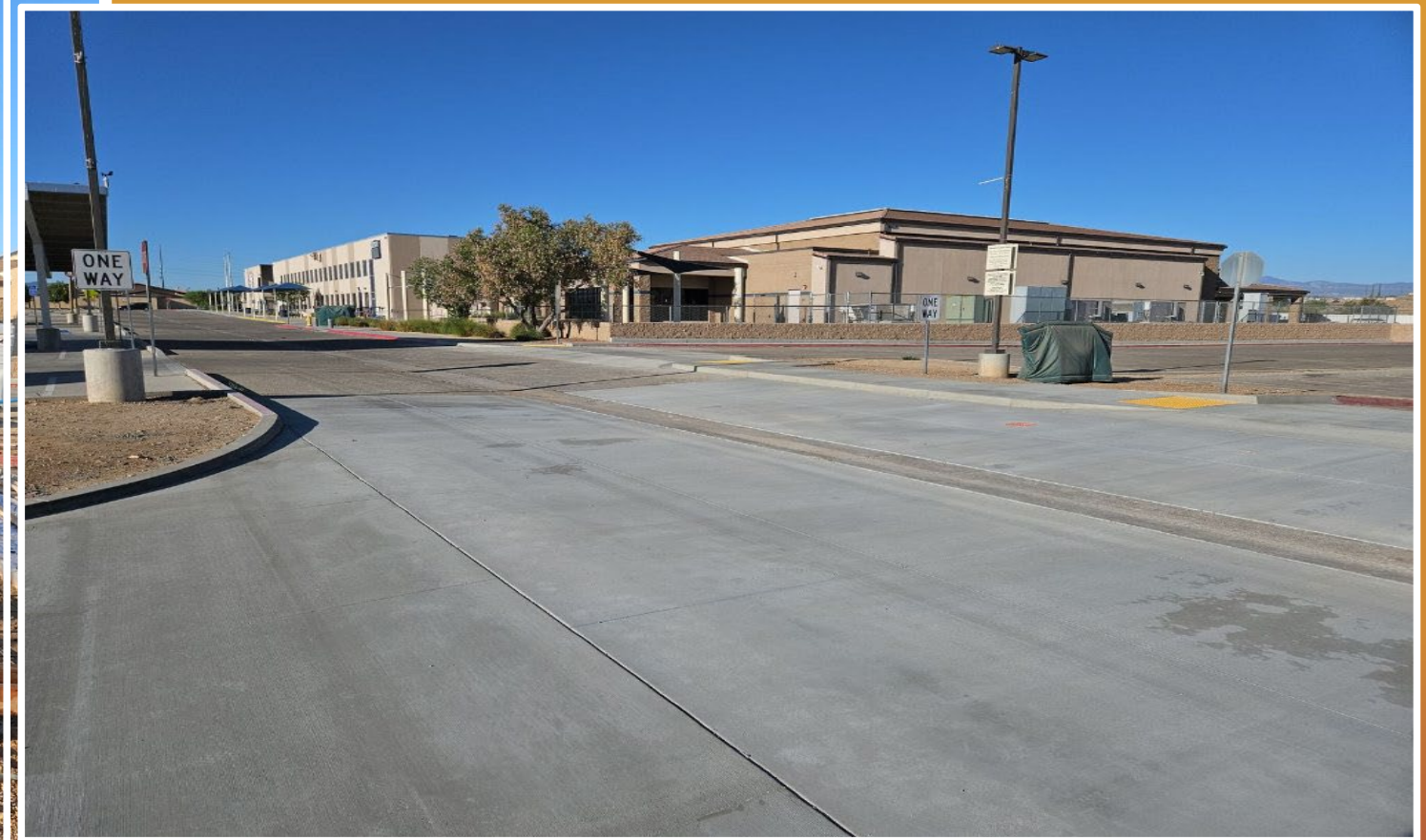
Making the Child Development Center more ADA Accessible
