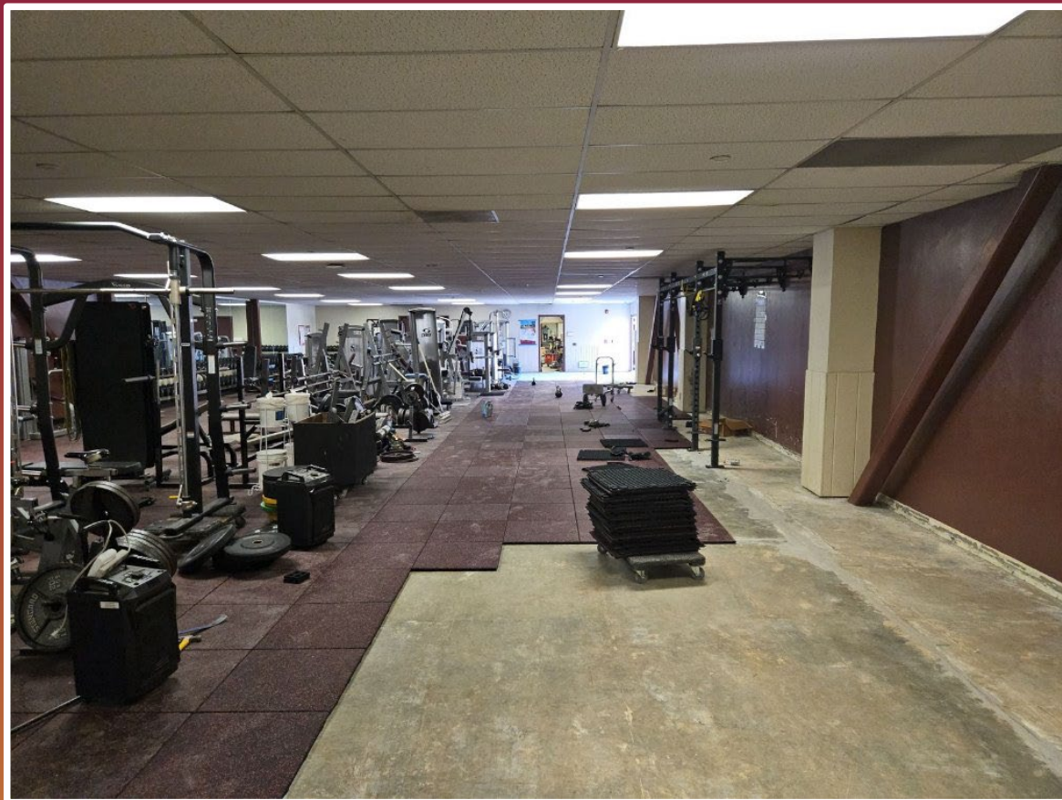
New flooring for the weight room
