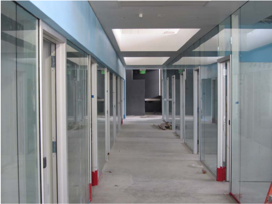
Faculty Office Corridor – November 23, 2011
