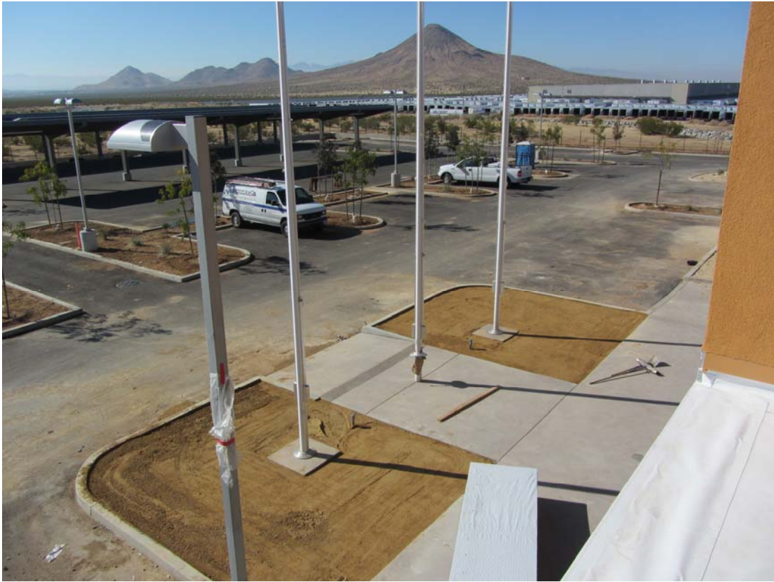
Main Parking Lot and Entrance Walkway – November 23, 2011
