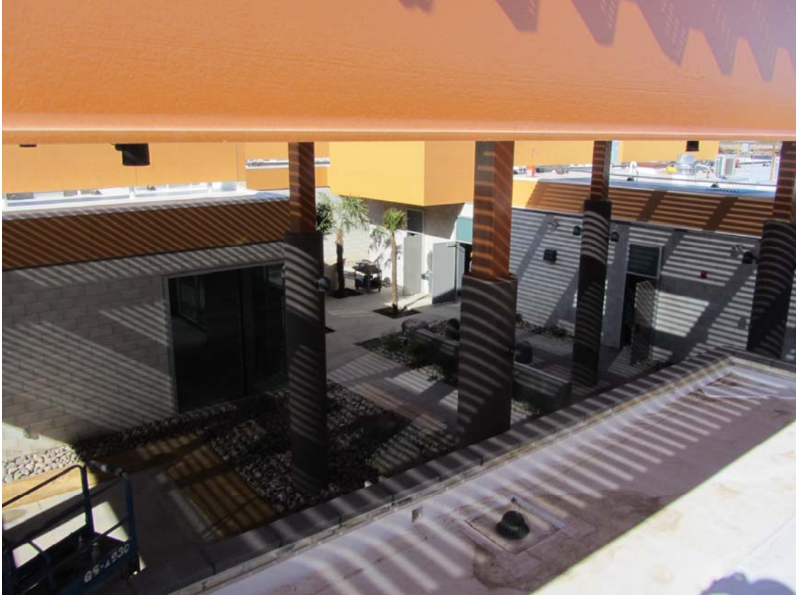
Covered Courtyard – November 23, 2011
