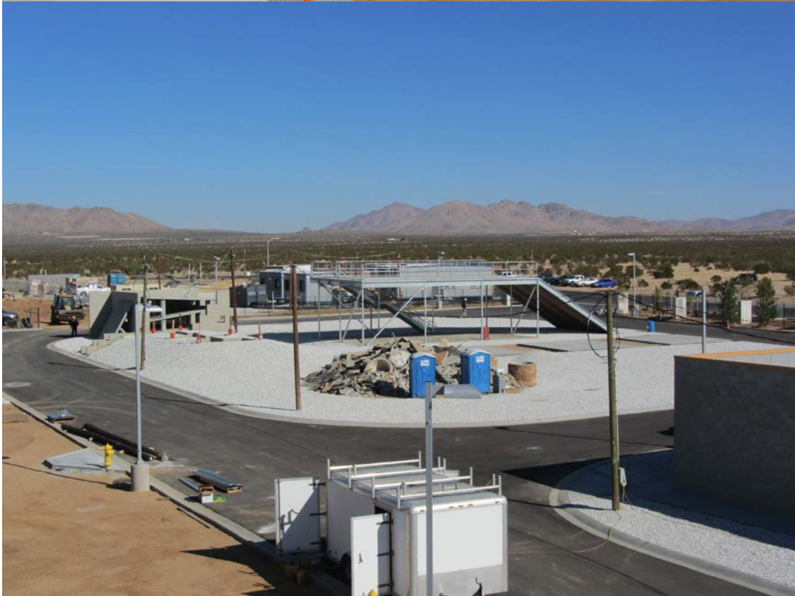
Prop Yard – November 23, 2011
