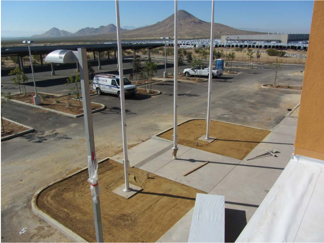
Main Parking Lot and Entrance Walkway – November 23, 2011
